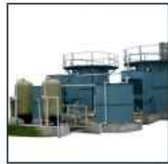
Effluent Treatment Plant
